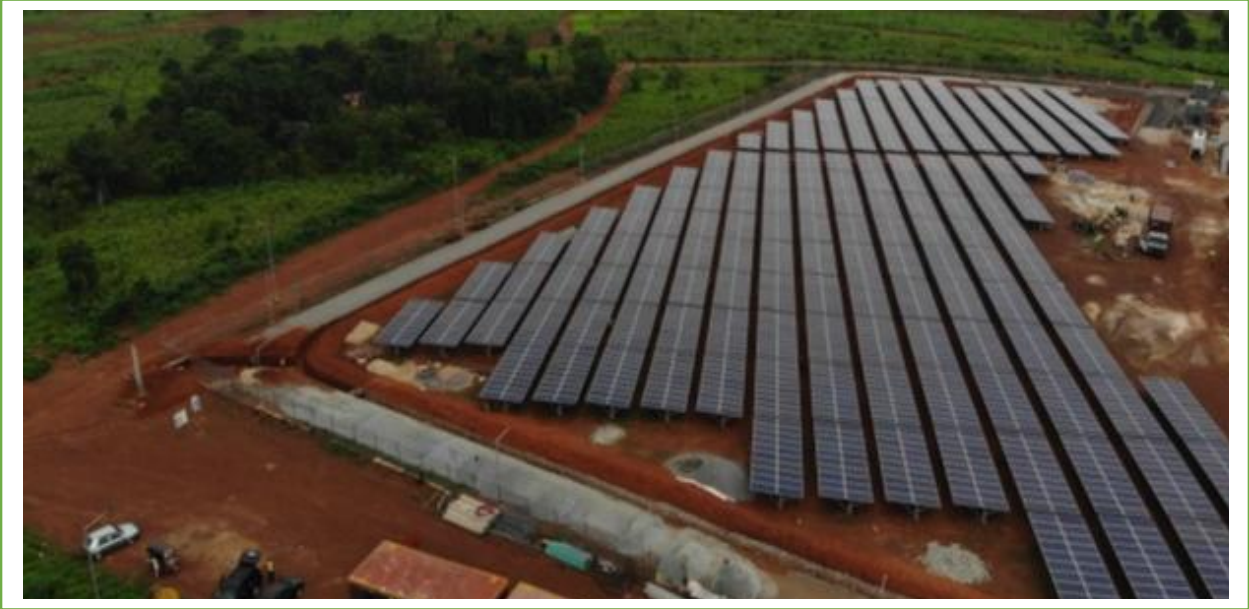
Figure 2: REA Solar Project FUNAI
