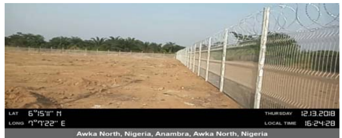
After Site Preparations (Fencing Completed)
