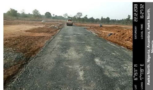
Internal Roads Preparations
