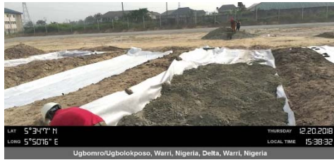
Equipment Foundation Works
