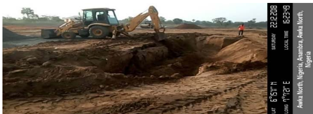
Equipment Foundation Works
