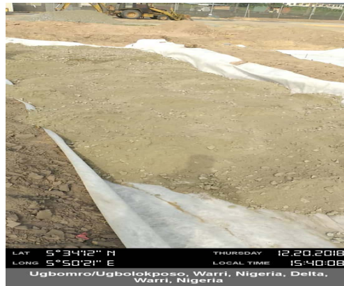
Site Internal Roads Preparations
