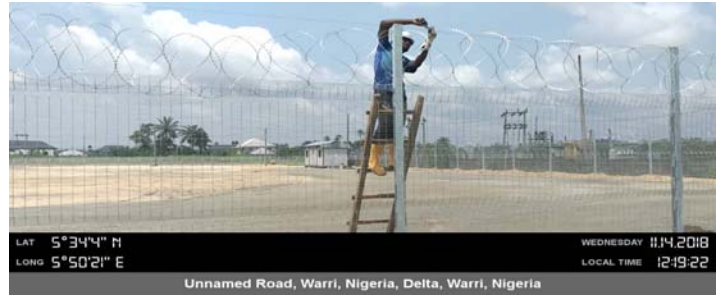
Installation of concertina wire on project site fence (Fencing Completed)
