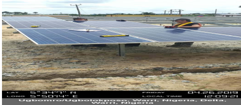
Solar Panels being mounted
